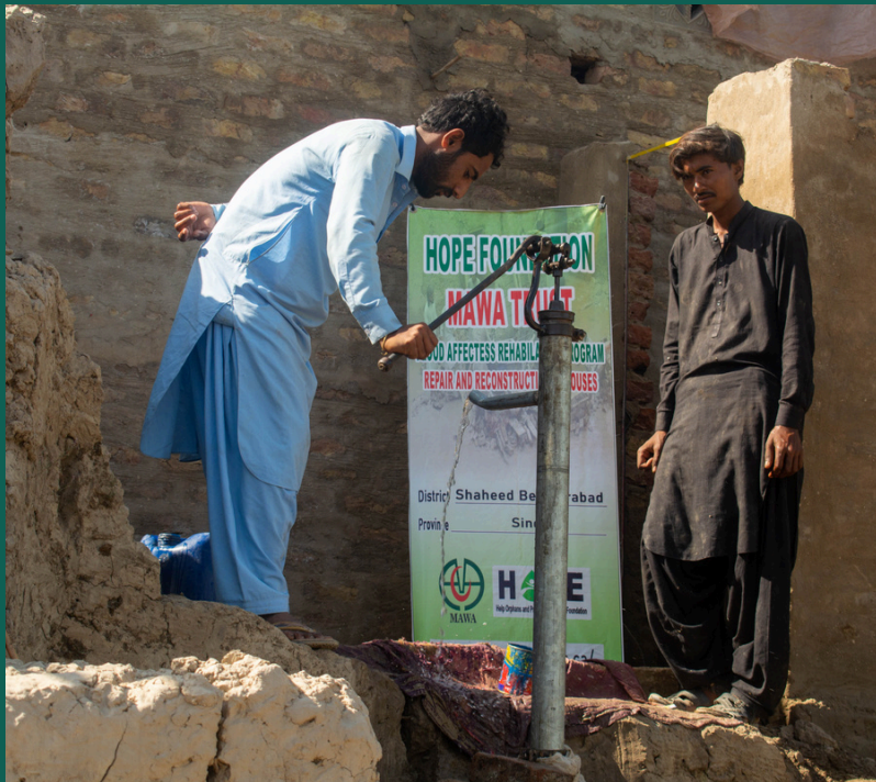
Construction of Hand Pump for Clean Water
